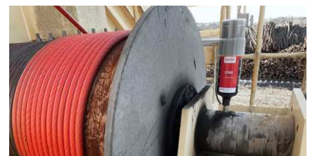
Lubrication of a crane cable pulley bearing
