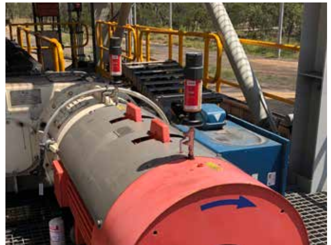
Application Electric motor Lubricator perma STAR VARIO 250cm 3 Installation kit Direct mount
