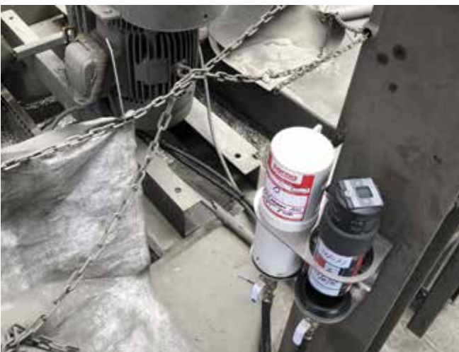
Application Sump pump Lubricator perma STAR VARIO 250 cm 3 Installation kit K230C
