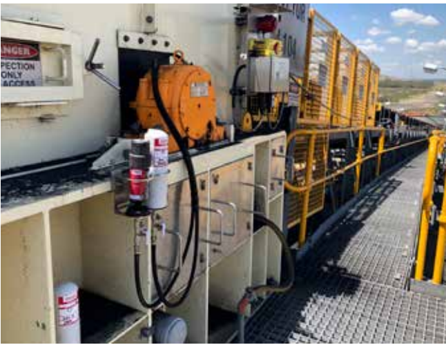
Application Conveyor pulley bearing and seal Lubricator perma STAR VARIO 250 cm 3 Installation kit K230C
