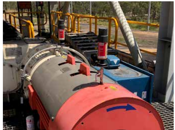
Application Electric motor Lubricator perma STAR VARIO 250 cm 3 Installation kit KDSV-708V
