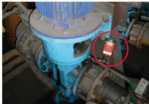
Fuel pump lubrication in the refinery process
