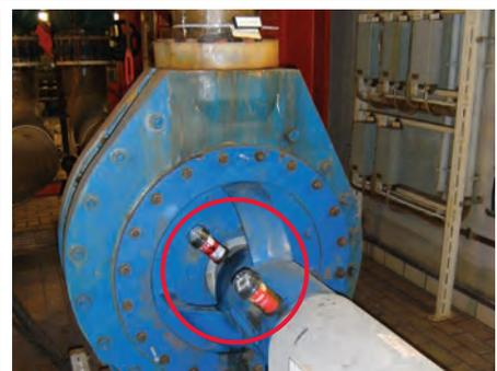
Drive shaft lubrication on a pump
