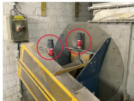
Pillow block bearing lubrication on a fan
