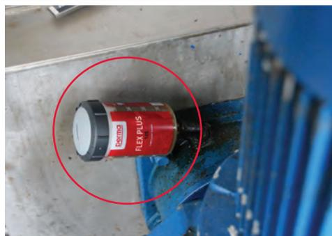
Bearing lubrication on a pump
