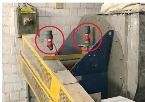
Lubrication of pillow block bearing on a fan
