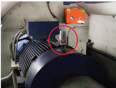
Automatic relubrication of the generator bearing
