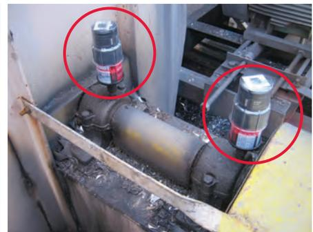
Lubrication of a fan drive shaft bearing
