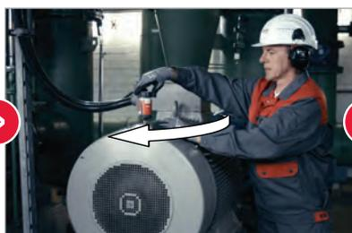
Screw lubrication system into lubrication point
