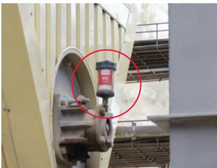
Flange bearing lubrication on the dedusting trough screw conveyor
